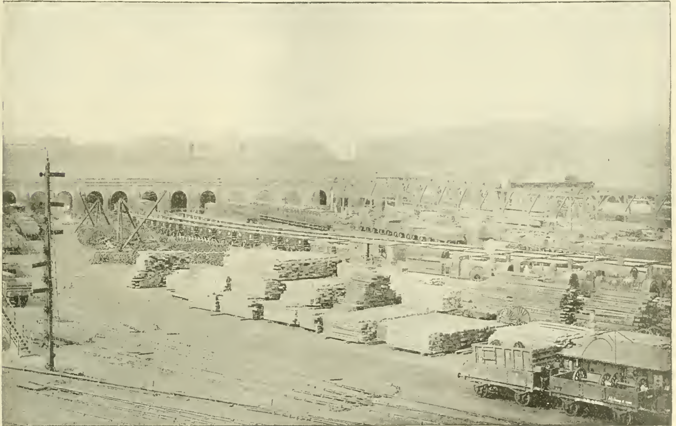
AS SEEN FROM ROOF OF THE PAINT SHOP.
